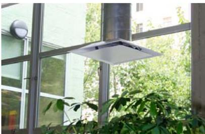
Therma-Fuser diffusers have the lowest pressure drop of any VAV terminal, allowing for low-pressure systems and low energy fan motors. And no energy is required to operate the diffuser's controls.
