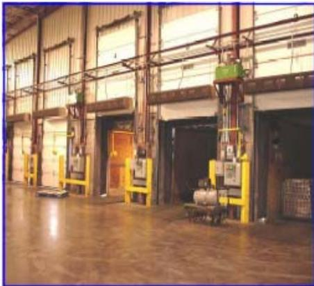
**Climate Control** is used in stopping cold or warm air from entering a climate controlled environment. It is available in unheated, electric, hot water, steam, indirect gas and direct gas heated versions. The **ETD** is commonly used in correctional facilities, trash compactors (odor control), beer distributors, walk in coolers, airports, and loading dock doors. As a general rule, the Climate Control unit has **less than a two year payback!!!**
